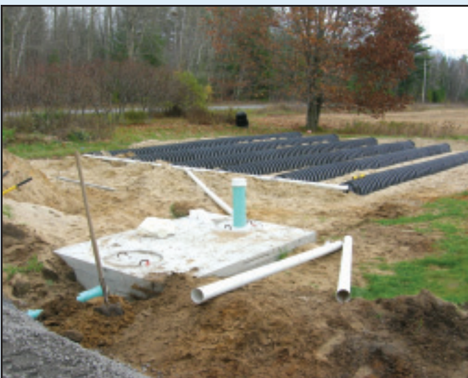
Leaching bed with gravelless trench technology.
