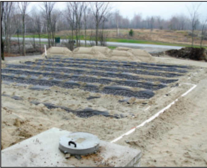
Leaching bed with perforated PVC drain pipes.
